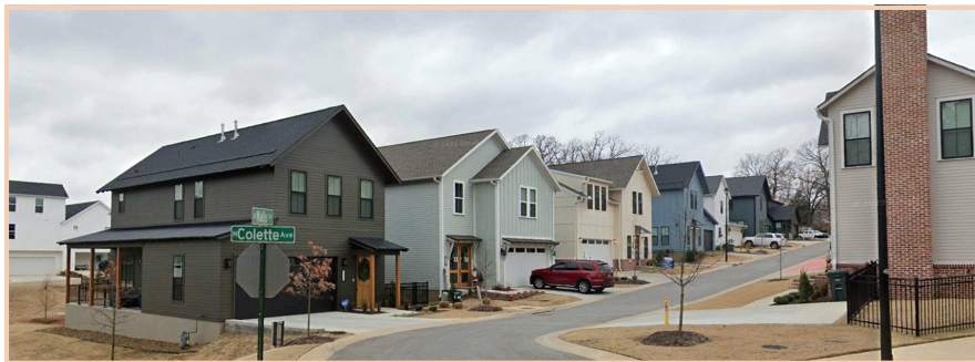
Gulley Grove Subdivision, Fayetteville, AR: With direct access to Gulley Park via dedicated central sidepath, this neighborhood near N. Old Wire Rd/Collette Ave features single-family homes on less than 0.10 acre lots, with approximately 1.5 acres dedicated to POA open space and recreation areas. This image/idea could inspire the mapped Neighborhood Residential areas.
