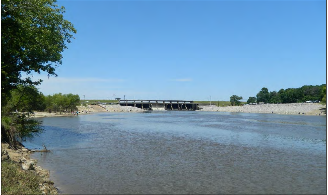
A view of the Ross Barnett Reservoir Dam north of the study area.
