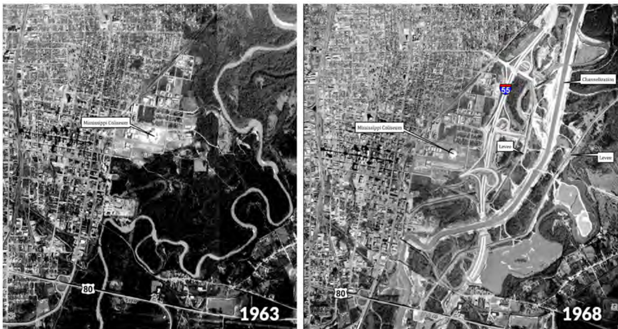
Figure 3-2. Pearl River Levee and Channelization Project Before and After.
