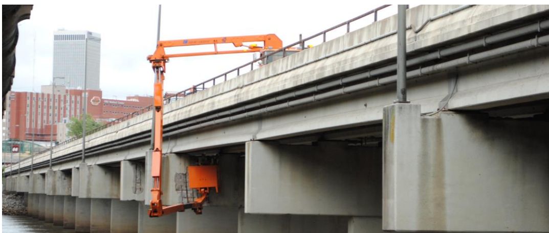
Figure 12 Snooper vehicle on the Southwest Boulevard Bridge
