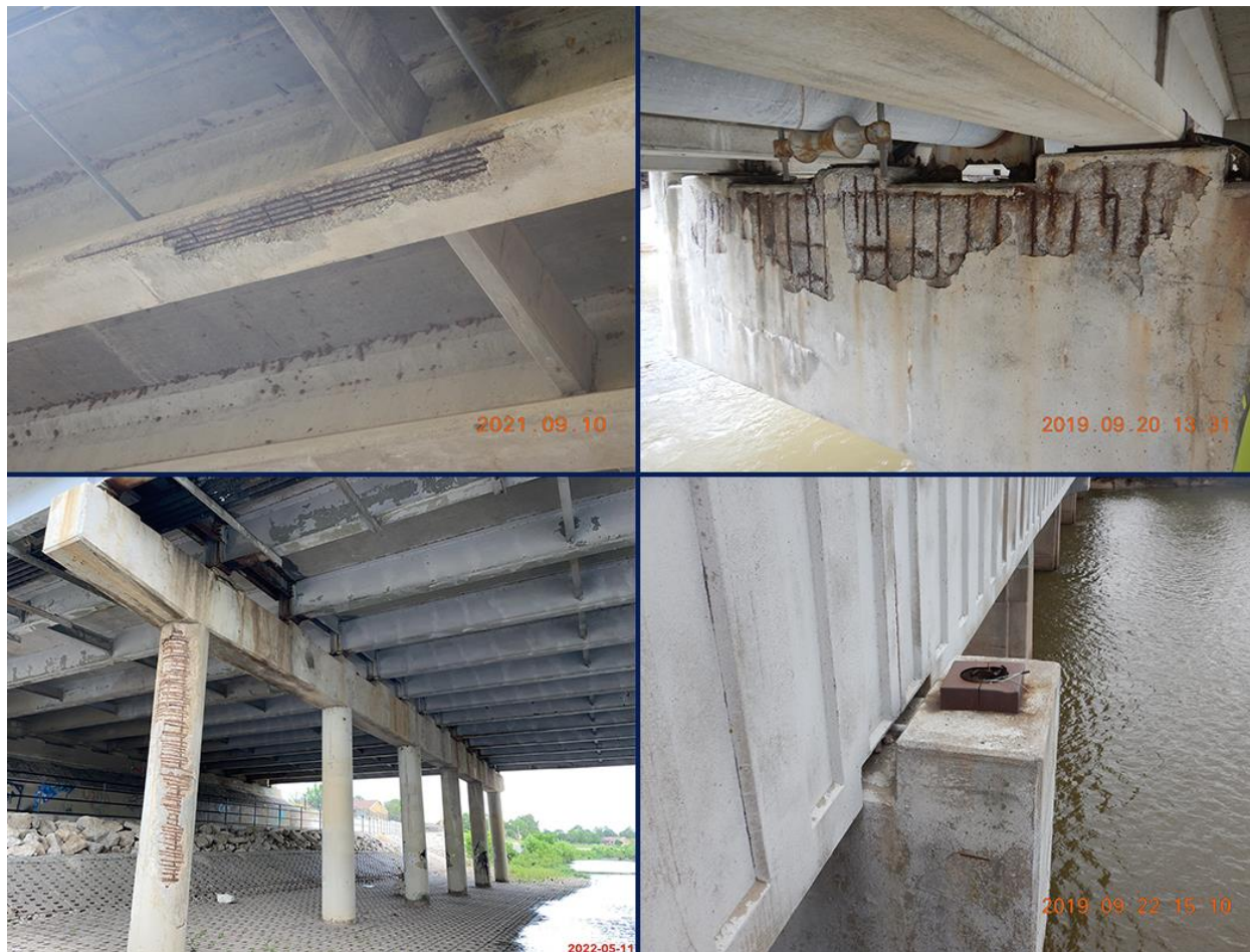
Figure 7 Deterioration Across all Four Bridges
