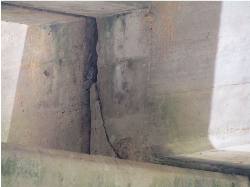
PHOTO 7 General Description BACK OF BEAM END SPALLED
