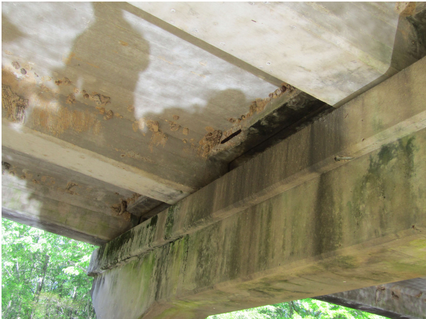
PHOTO 8 General Description DROP SLAB SPALLED
