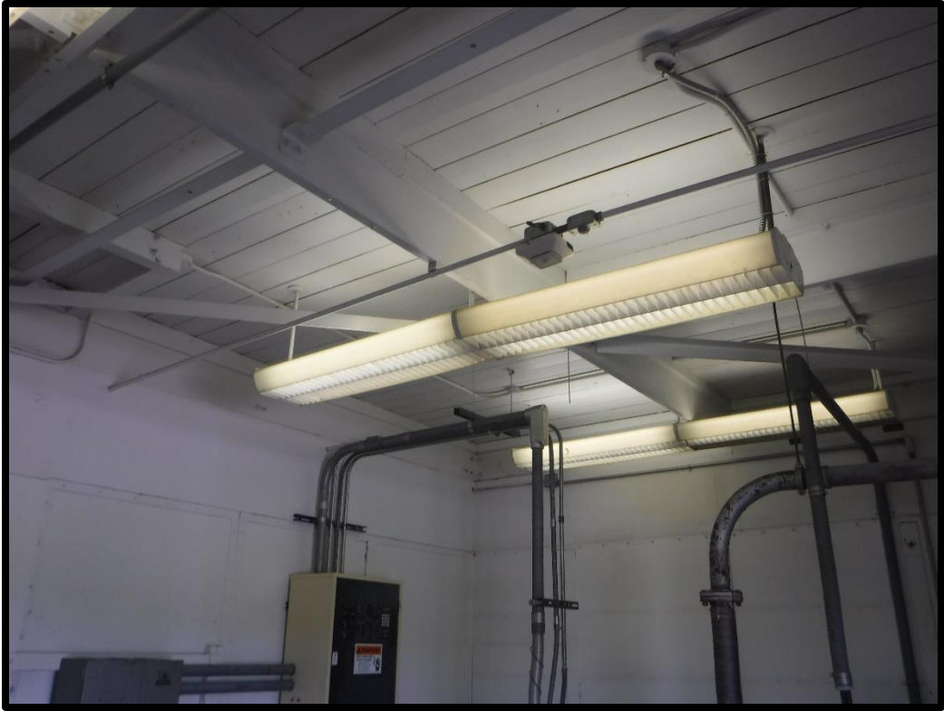
Figure 14. View of Generator Room ceiling of Little Rock VORTAC building
