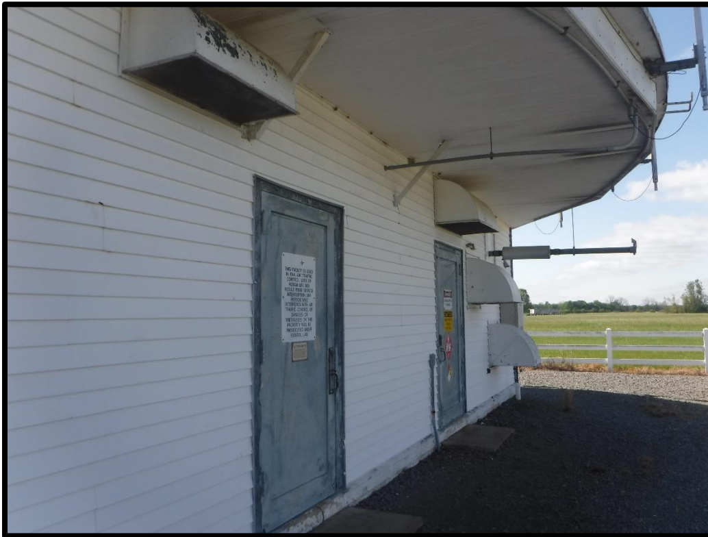
Figure 7. View of Western façade of Little Rock VORTAC building (facing south-southeast)
