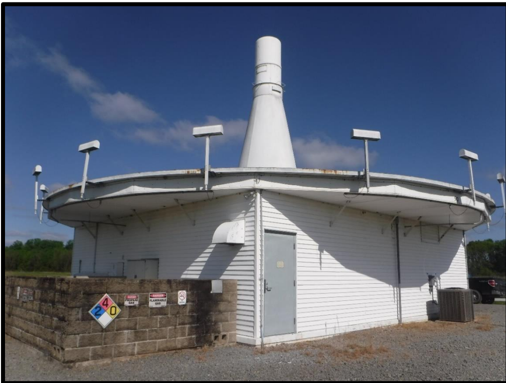
Figure 5. View of Southern and Eastern façades of Little Rock VORTAC building (facing northwest)
