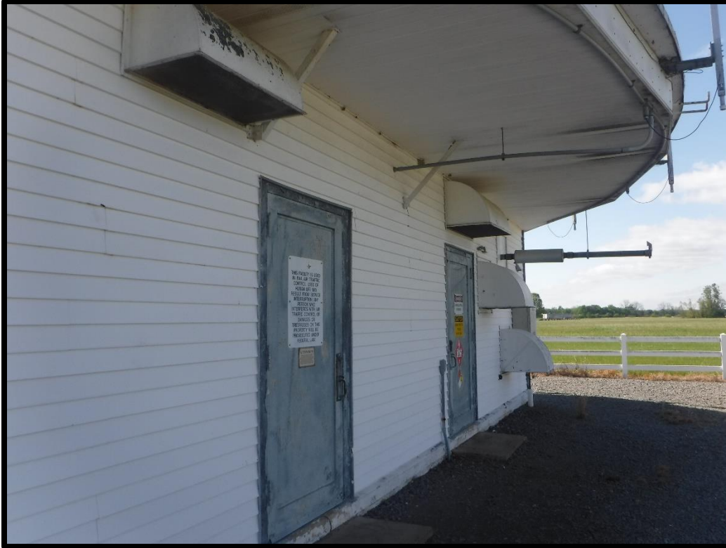
Figure 8. View of Western façade of Little Rock VORTAC building (facing south-southeast)
