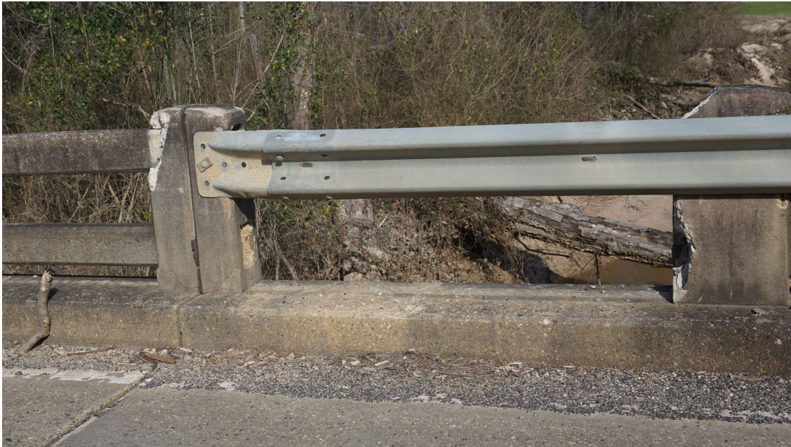
PHOTO 13 Deck Description BRIDGERAIL DAMAGE AT SPAN 6 NORTH SIDE.
