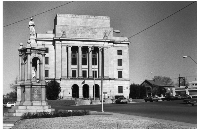
U.S. Courthouse and Post Office in Texarkana (Photo by John Gill) Modern Era (1968 - the Present)
