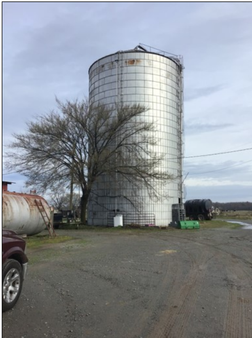
Figure 3. Grain silo near proposed VOR site.
