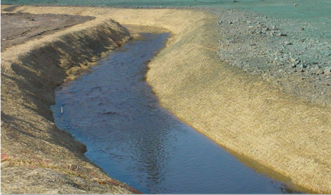
Photograph CS-3 – Example of Erosion Control Blanket
