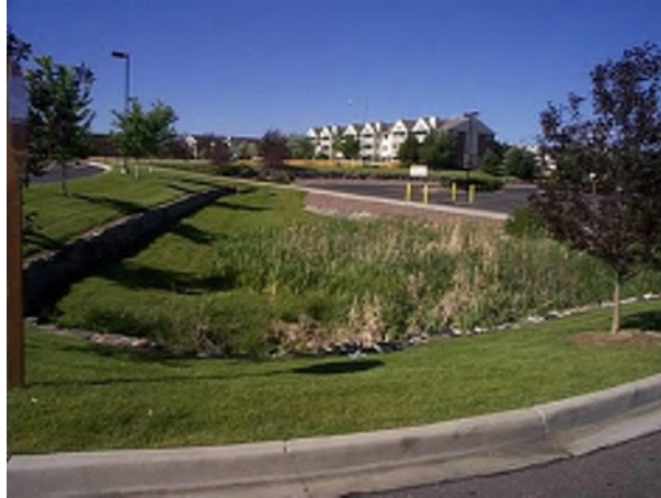
Photograph WQ-1 – Example of a dry detention basin. Properly designed and maintained an extended dry detention basin can be a site amenity.
