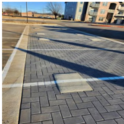
Photograph WQ-6 – Example of Permeable Pavers.
