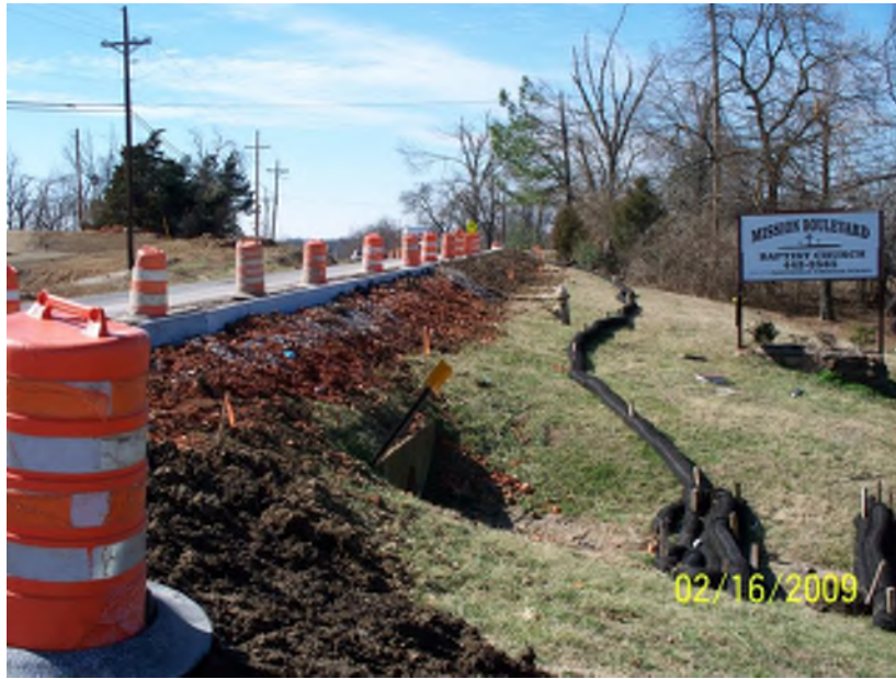
Photograph CS-7 – Example of Fiber Roll/Wattle
