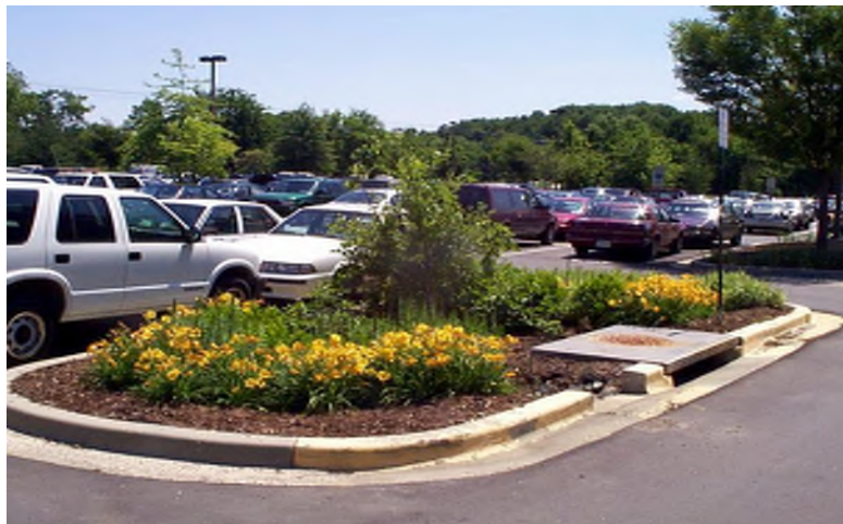
Photograph WQ-13 – Example of a Porous Detention Island. This porous detention island is designed to reduce runoff rates and volumes and pollutant loading.
