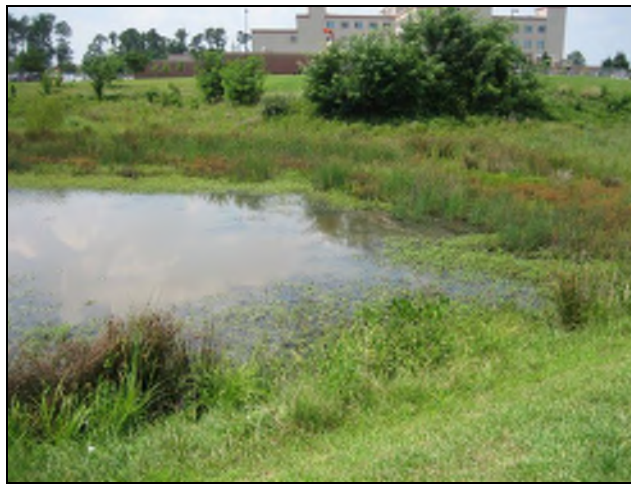
Photograph WQ-3 – Example of a Constructed Wetland Basin.
