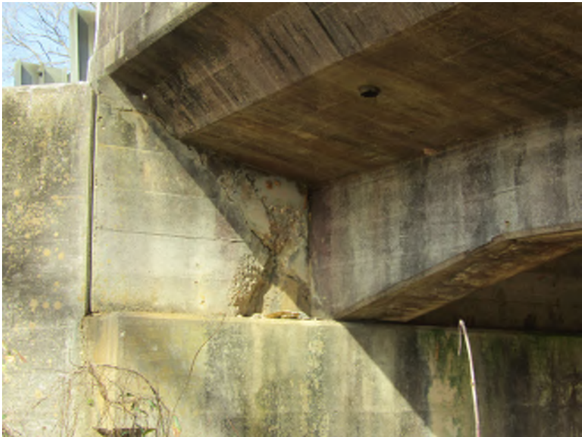
PHOTO 8 General Description DIA SPALLED
