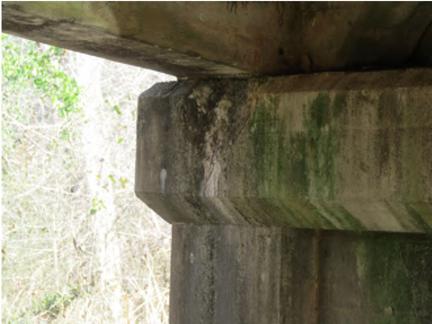
PHOTO 7 General Description CAP SPALLED
