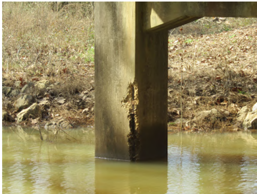
PHOTO 10 General Description SPALL COLUMN 2 BENT 2
