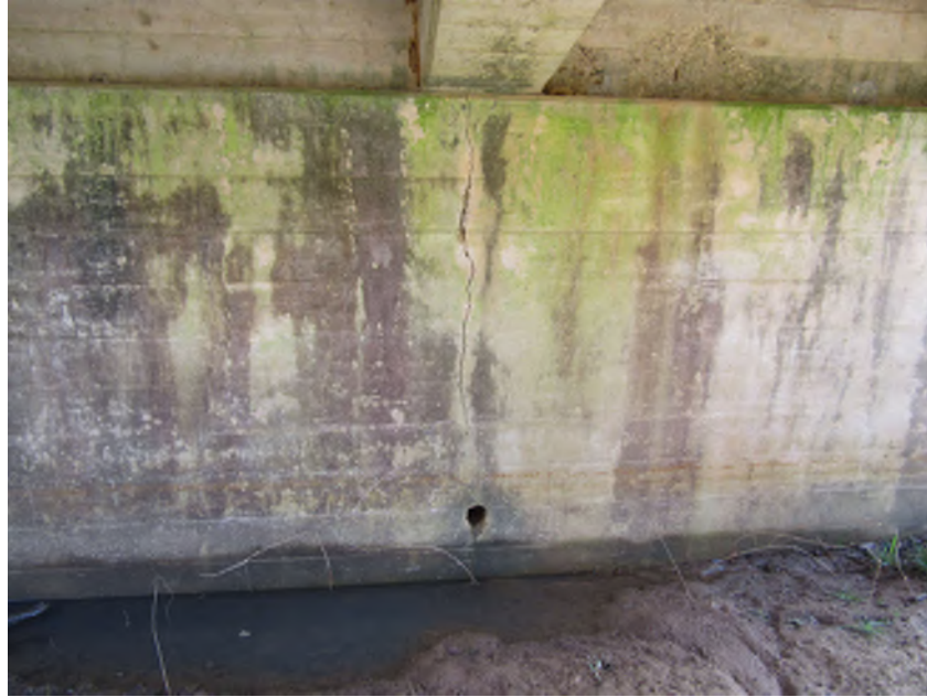
PHOTO 11 General Description CRAK IN ENDWALL
