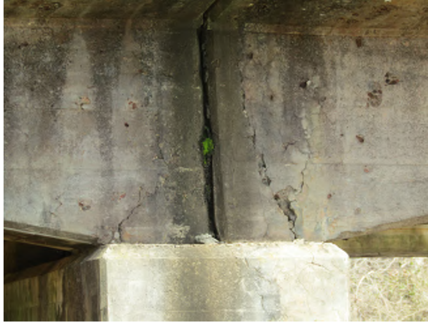
PHOTO 5 General Description BEAM END CRACKED
