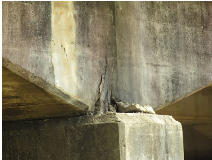
PHOTO 6 General Description BEAM END CRACKED
