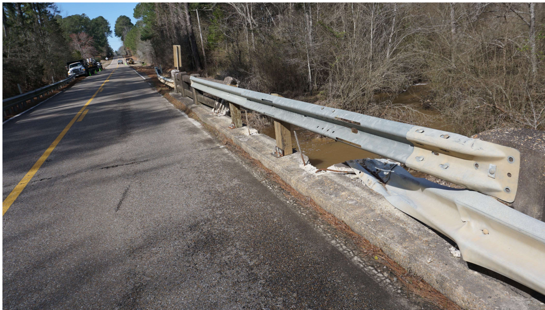
PHOTO 2 Deck Description DAMAGE TO WEST BOUND RAIL
