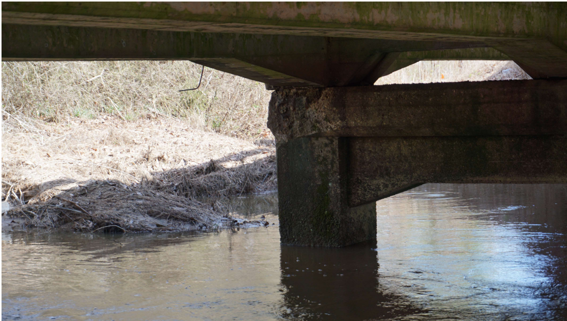
PHOTO 8 Substructure Description SPALL AT FACE OF CAP AT BENT 2, SPALL AT NE CORNER.
