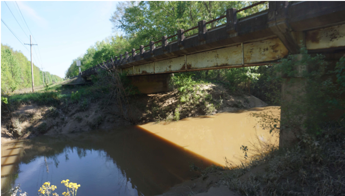
PHOTO 10 General, Channel Description UPSTREAM
