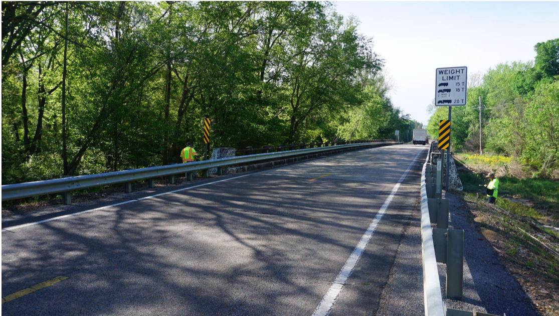
PHOTO 13 General, Approach Description CENTER LINE SOUTH.
