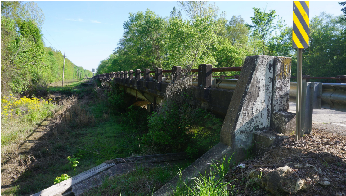
PHOTO 3 General, Superstructure Description ELEVATION WEST
