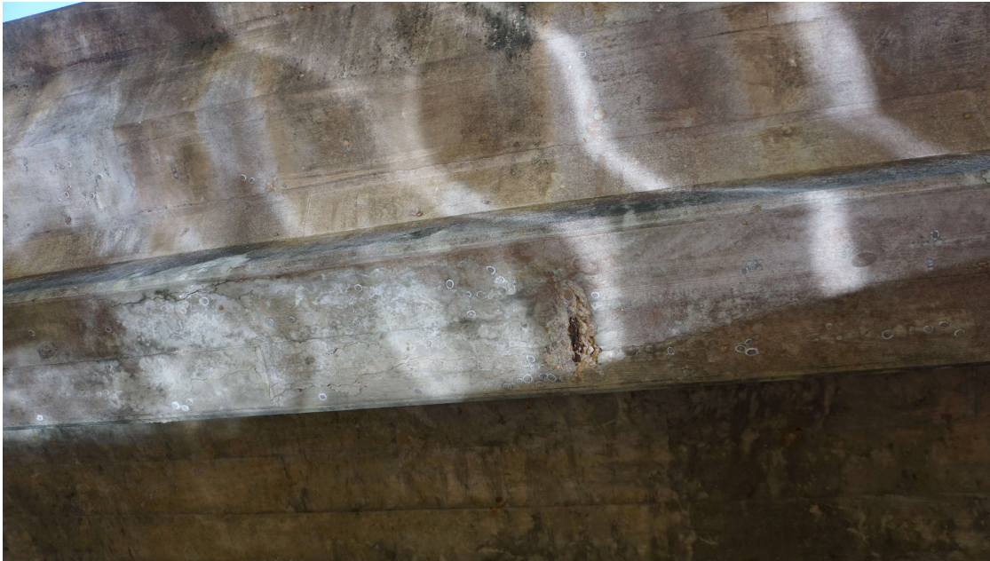
PHOTO 7 Superstructure Description SPALL AND DELAM BEAM 3 SPAN 2 BOTTOM OF BEAM 4'X1'. VC'S AT R/C BEAMS
