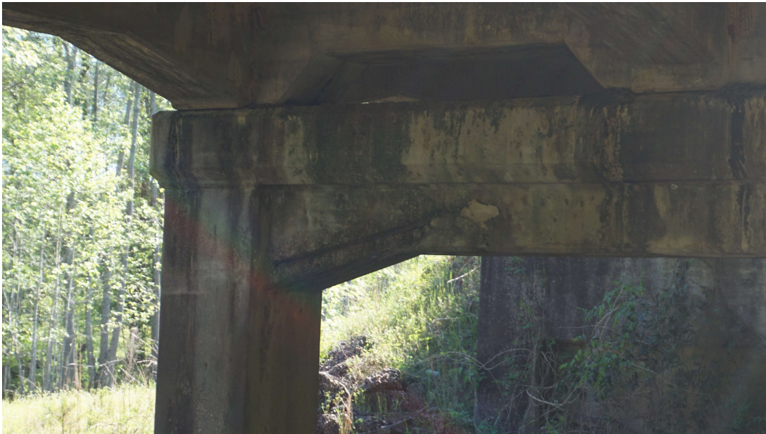
PHOTO 6 Substructure Description B-3 SPAN 2, SPALLS IN CAP.
