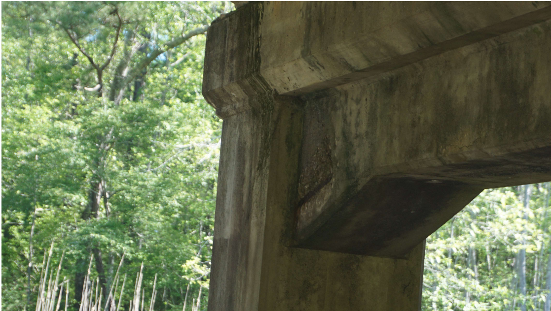
PHOTO 5 Substructure Description B-2 SPAN 1, SPALL WITH EXP. REBAR 1' X1' FACE OF CAP
