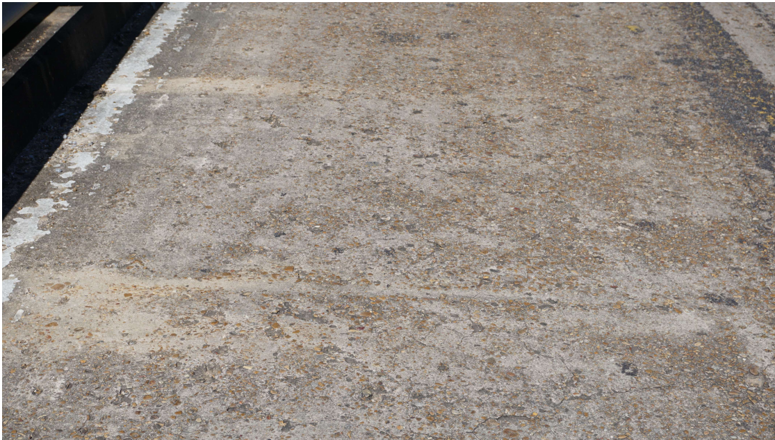
PHOTO 10 Deck Description MOD. DECK SCALING. SEVERAL POP OUTS
