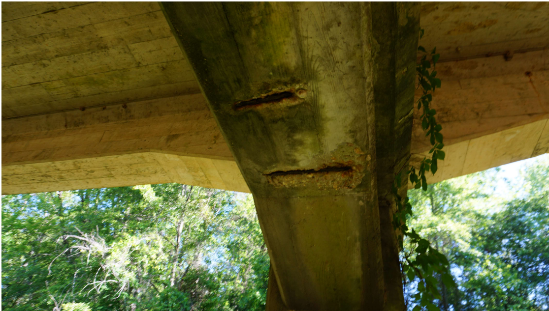
PHOTO 7 Substructure Description REBAR EXP. AT BOTTOMOF CAP AT BENT 4, 2' X 2'.
