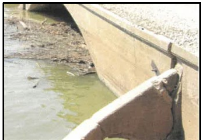
Figure 4: Cracked Wingwall
