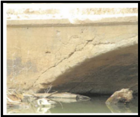
Figure 3: Load cracks on Hunnewell Bridge
