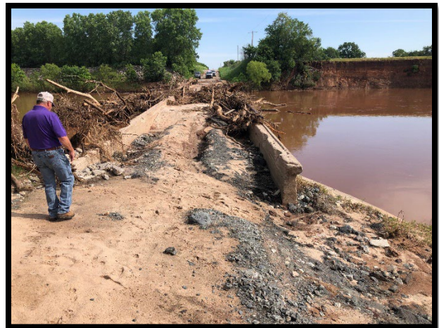
Figure 2: Driving surface erosion due to flooding, 2019
