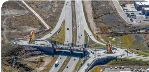
I-25/Dillon Drive Interchange Improvements City of Pueblo, CO
