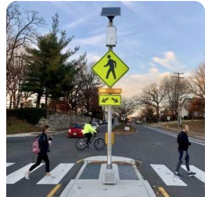
RRFB • Arlington County, VA
