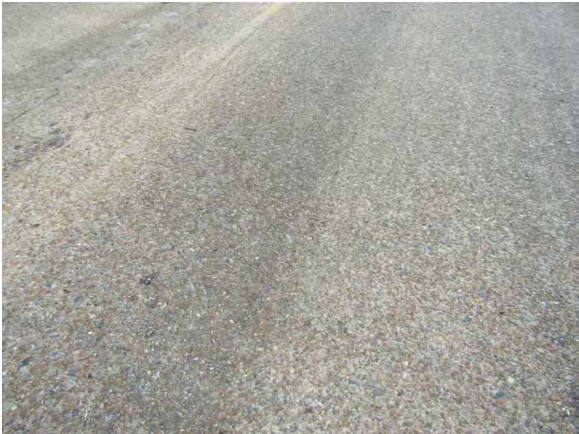
PHOTO 4 General Description LIGHT DECK SCALING
