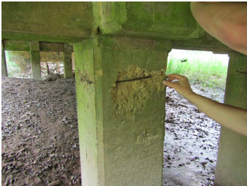
PHOTO 18 General Description EXP REINFORCEMENT AT ALL PILES BENT 2
