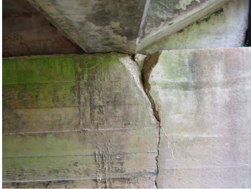
PHOTO 9 General Description VC&#39;S IN ABUTMENT WALL
