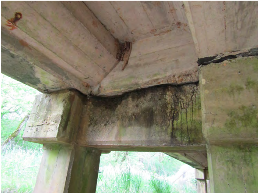
PHOTO 21 General Description CAP SPALLED AT BENT 3 SPAN 4
