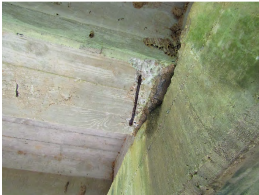
PHOTO 10 General Description B-3 BEAM 3 SPAN 3 EXP REBAR IN BEAM END
