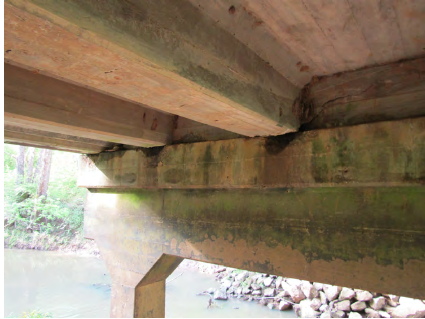
PHOTO 7 General Description BENT 5 SPAN 5 SPALL TO FACE OF CAP UNDER BEAMS 3,4,5
