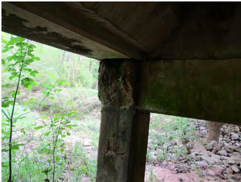
PHOTO 20 General Description CAP SPALLED AT BENT 3 SPAN 2
