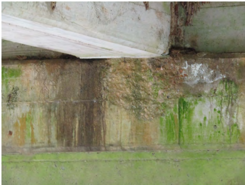
PHOTO 12 General Description CAP SPALLED UNDER BEAMS 1 AND 3 BENT 4
