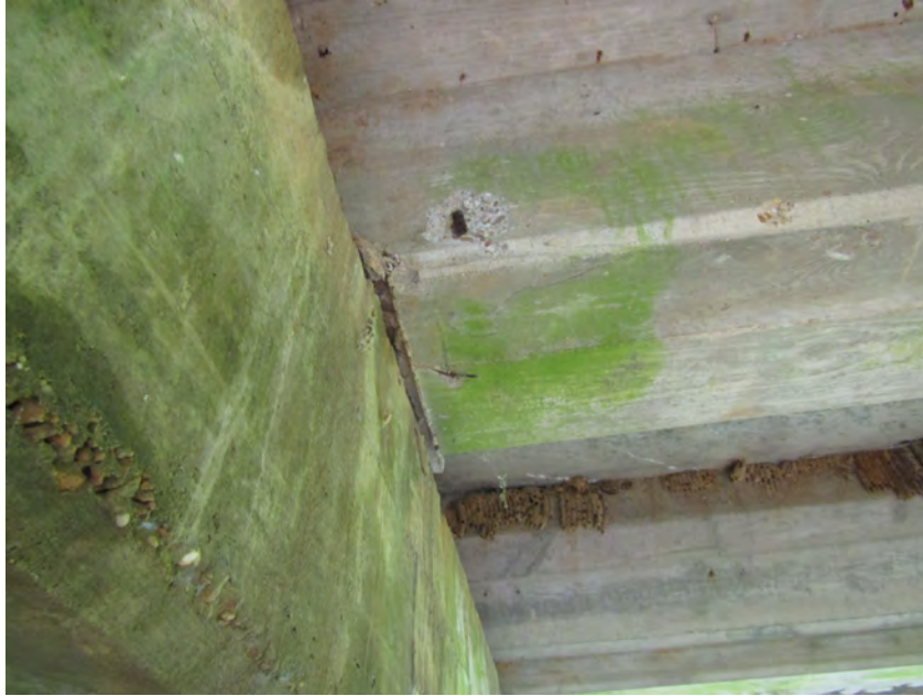
PHOTO 11 General Description BEAM SPALLED BENT 3
