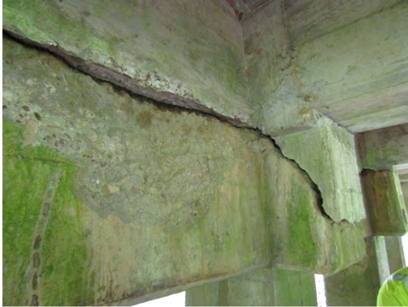
PHOTO 19 General Description DELAM ON CAP UNDER BEAMS 3 AND 4 BENT 2
