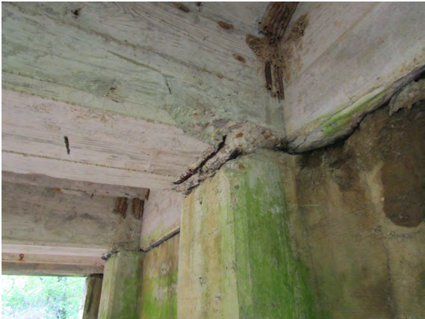
PHOTO 22 General Description BEAM 3 SPAN 3 EXP REBAR
