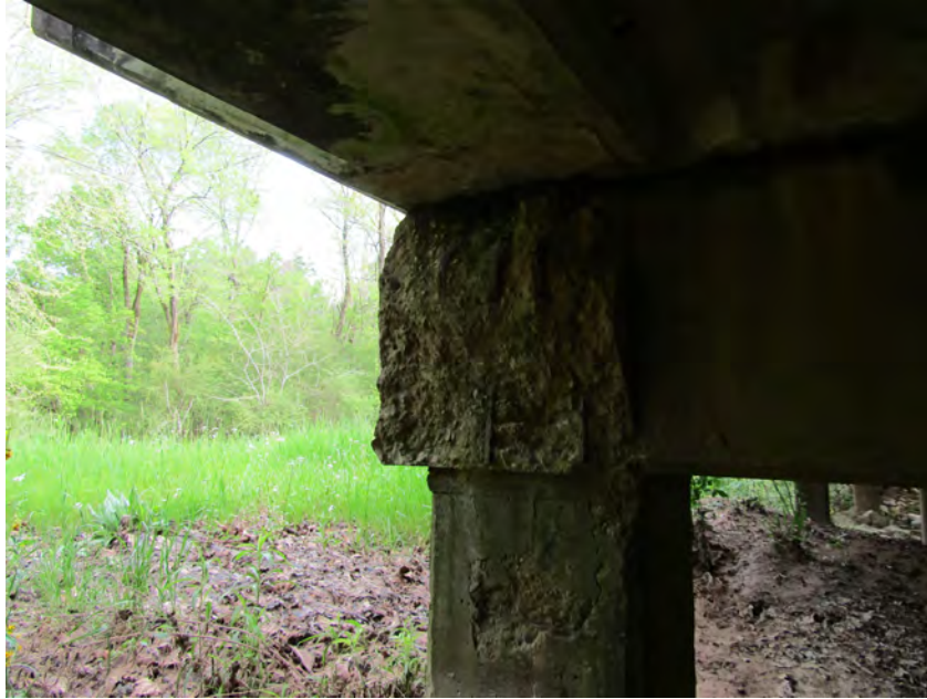
PHOTO 17 General Description CAP SPALLED AT BENT 2 SPAN 1 2&#39;X1&#39; UNDER BEAM 1
