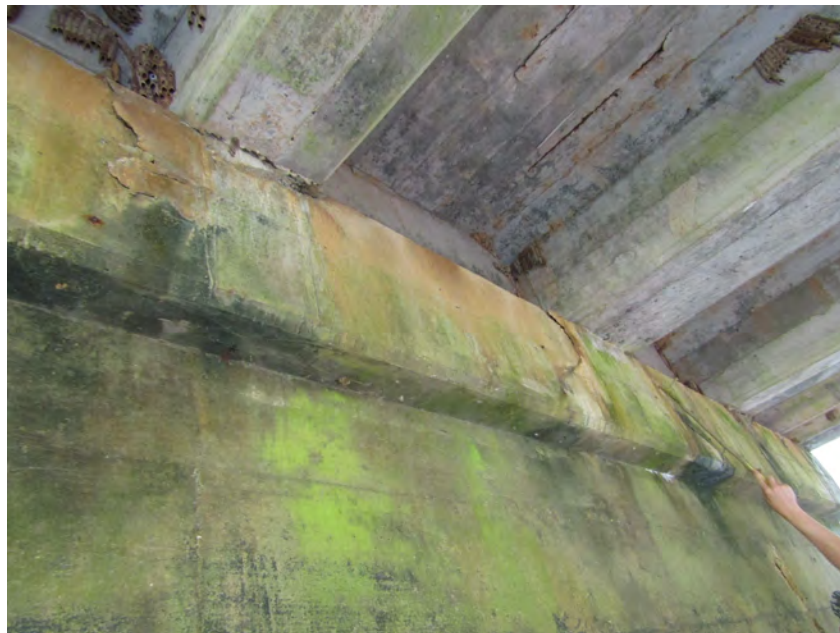
PHOTO 8 General Description BENT 5 SPAN 4 DELAMS FACE OF CAP
