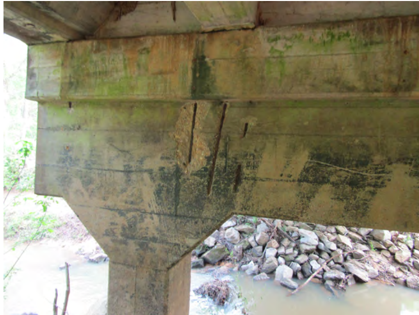
PHOTO 23 General Description EXP REBAR FACE OF CAP BENT 4
