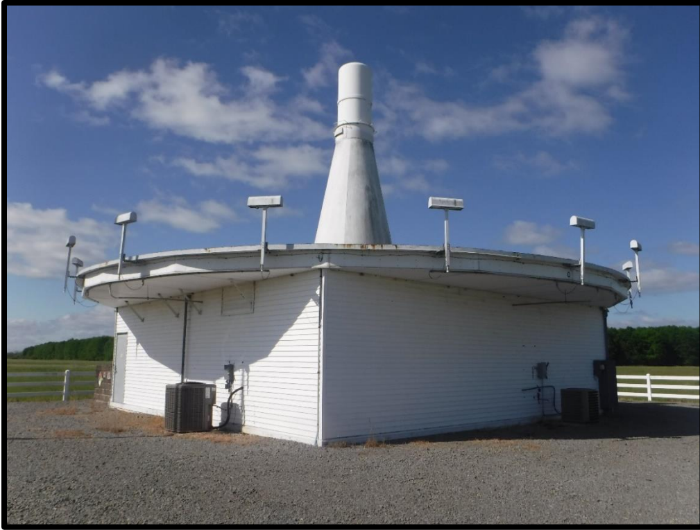
Figure 6. View of Eastern and Northern façades of Little Rock VORTAC building (facing southwest)
