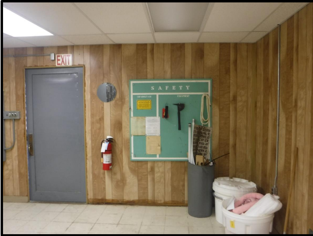
Figure 10. View of entryway leading to Equipment Room of Little Rock VORTAC building
