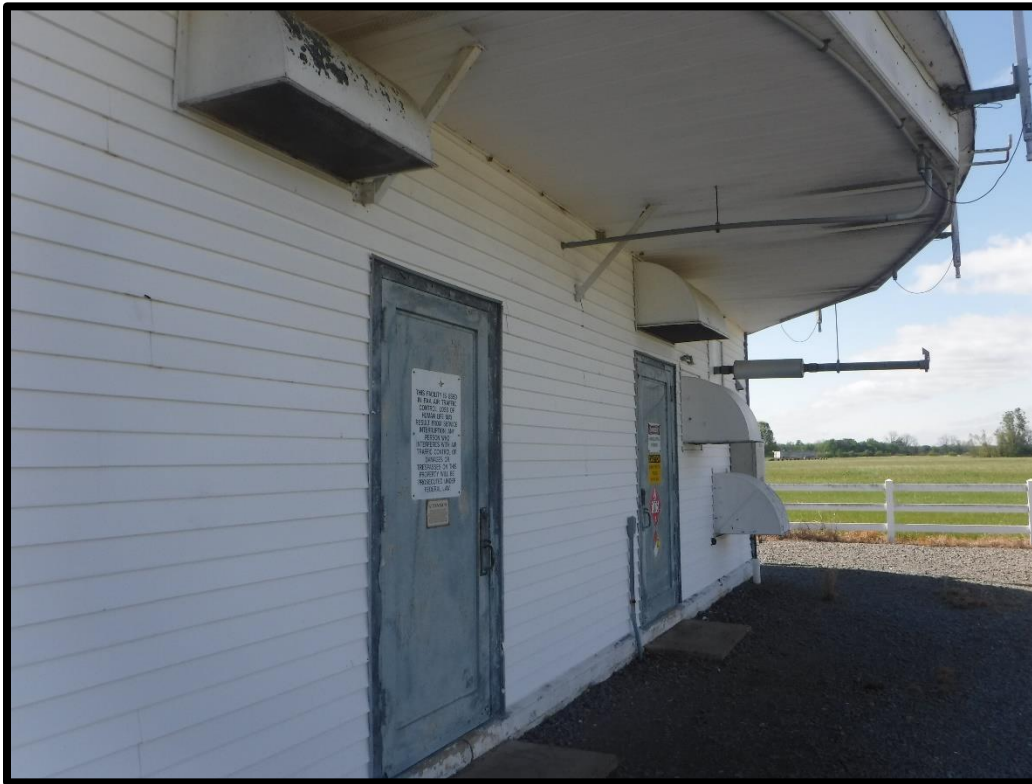
Figure 7. View of Western façade of Little Rock VORTAC building (facing south-southeast)
