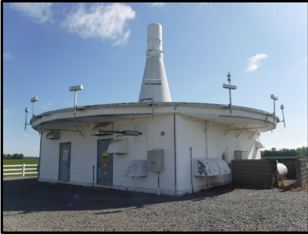
Figure 4. View of Western and Southern façades of Little Rock VORTAC building (facing northeast)
