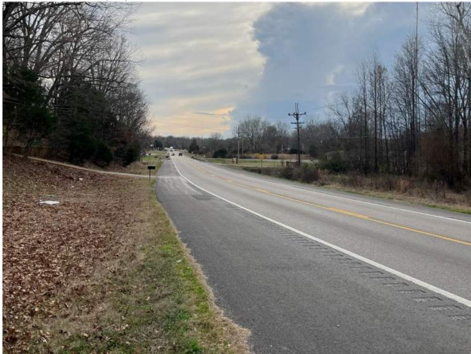
Photo 16: View facing south toward location where the eastern project roadways would tie into Highway 67. (Photo taken on March 4, 2024.)
