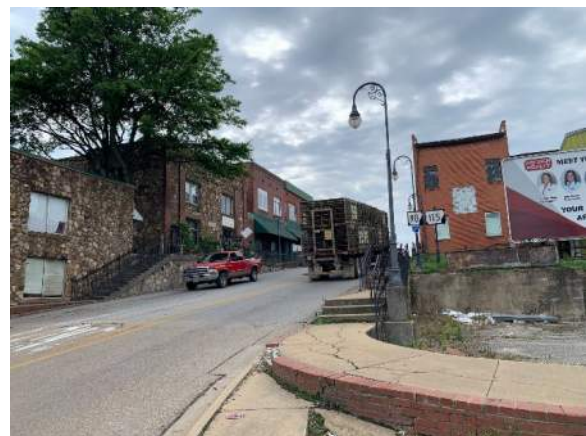
Figure 3: Steep incline on Hwy 90
