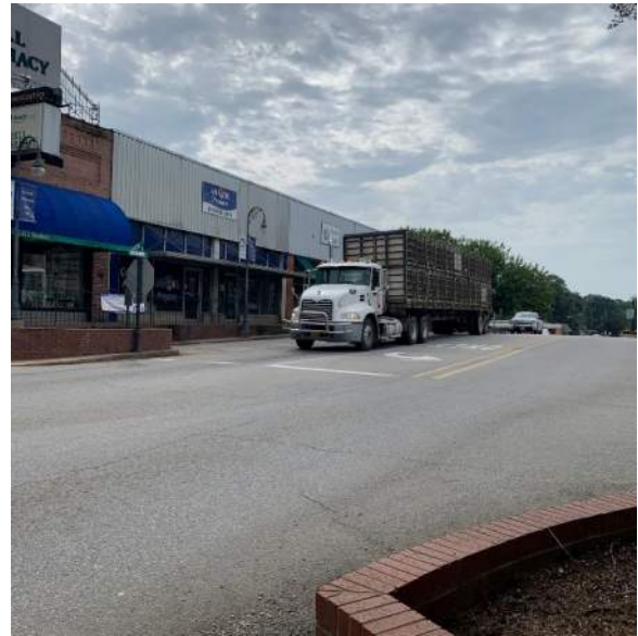
Figure 5: Narrow Lanes on Hwy 90
