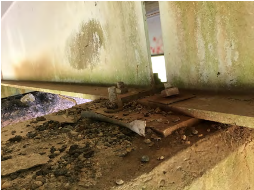
PHOTO 32 Superstructure Description Typical bearings
