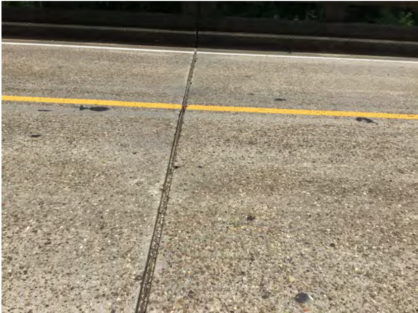
PHOTO 27 Deck Description Typical intermediate joints.
