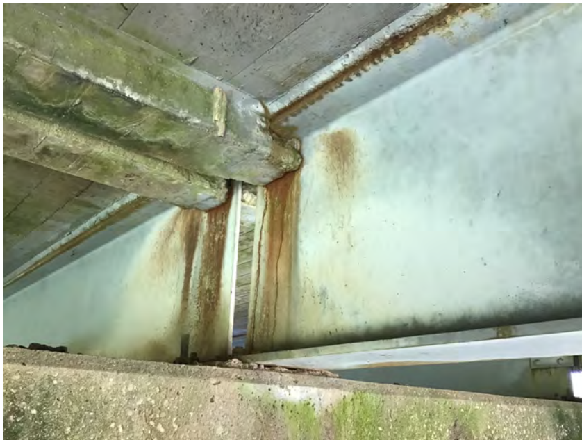
PHOTO 36 Superstructure Description Typical girder ends.
