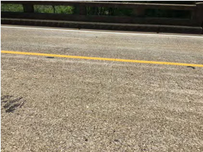
PHOTO 28 Deck Description Typical cracks in deck
