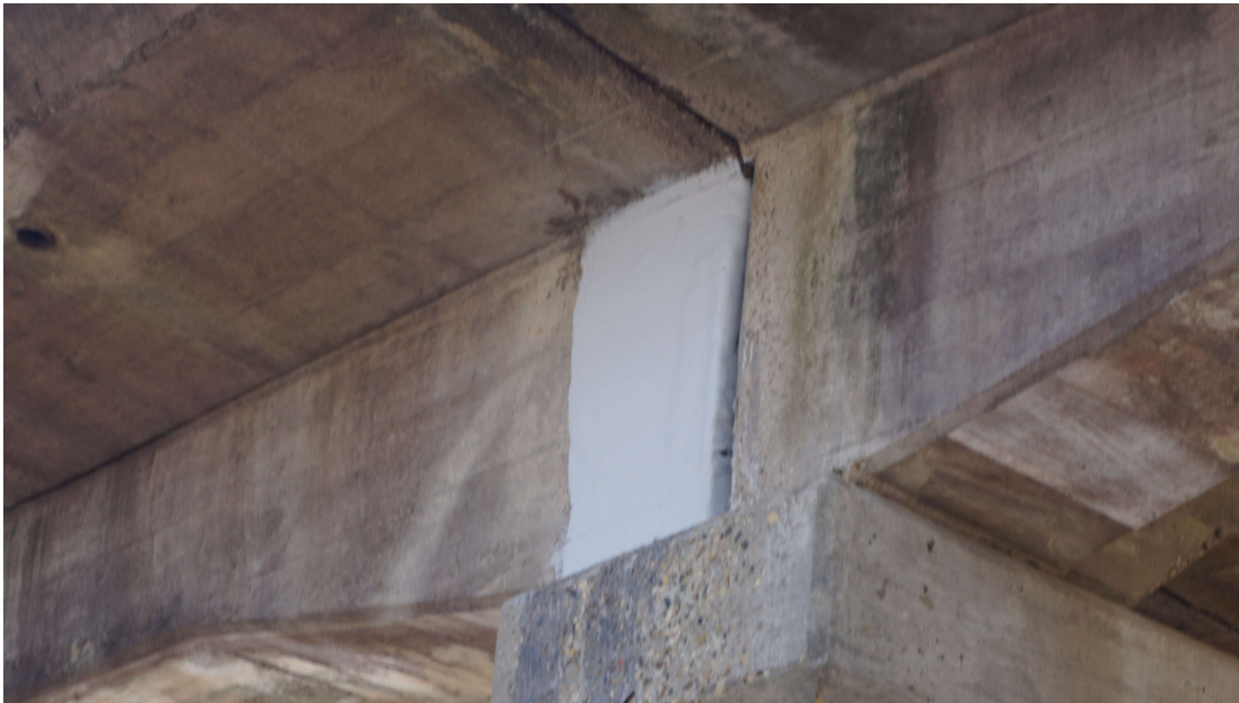
PHOTO 4 Superstructure Description BEAM END REPAIR B-2
