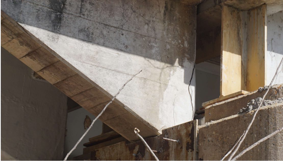
PHOTO 7 Superstructure Description B-8 SPAN 8 BEAM 3 NOT REPAIRED, CRACK.
