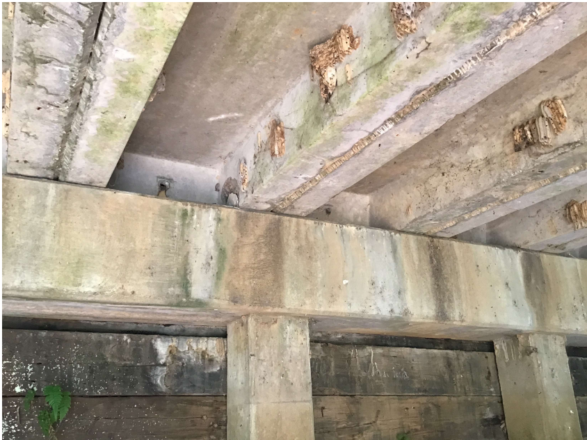
PHOTO 8 Superstructure Description Minor spall in channel beam above pile 6 bent 1
