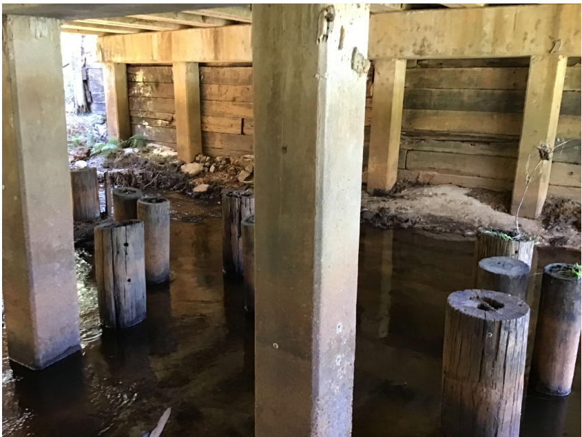
PHOTO 6 Substructure Description South abutment
