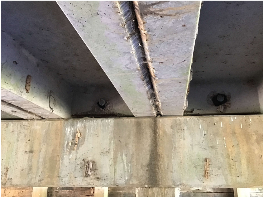
PHOTO 7 Superstructure Description Typical spalls with exposed rebar
