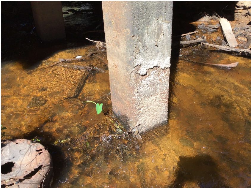
PHOTO 10 Substructure Description Typical waterline abrasion on piles bent 2
