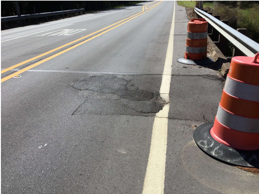
PHOTO 19 Approach Description Settlement at Northwest corner of bridge
