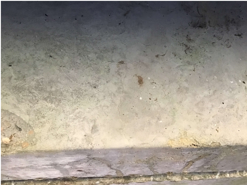
PHOTO 4 Superstructure Description Typical cracks in channel beams
