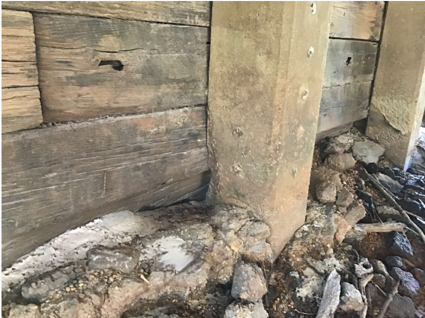
PHOTO 15 Substructure Description Spall in pile 5 of bent 1
