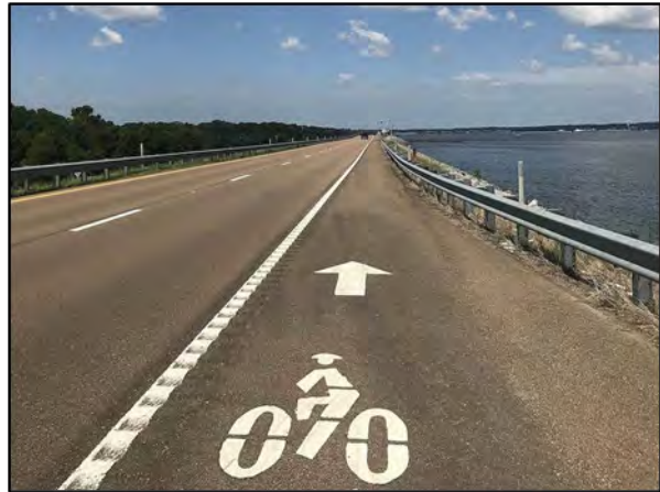
Figure 7 - View of the existing, unprotected bike lane on the Dam.
