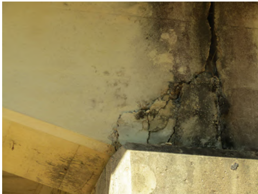
PHOTO 4 General Description back of beam end spalled
