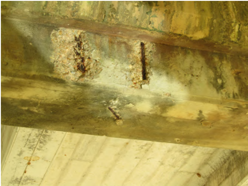
PHOTO 2 General, Substructure Description exposed rebar in face of cap
