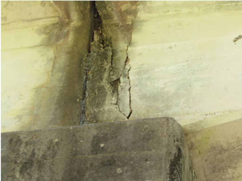
PHOTO 1 General, Superstructure Description back of beam end spalled
