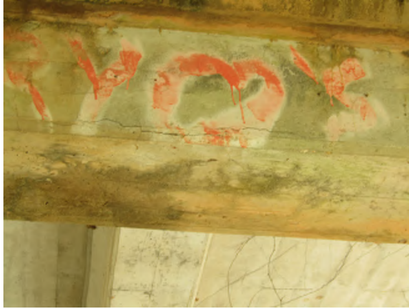
PHOTO 3 General, Superstructure Description horizontal crack in beam
