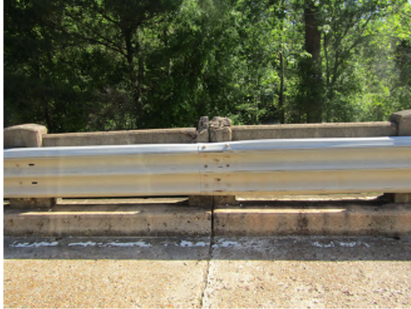
PHOTO 13 General Description top of bridgerail spalled
