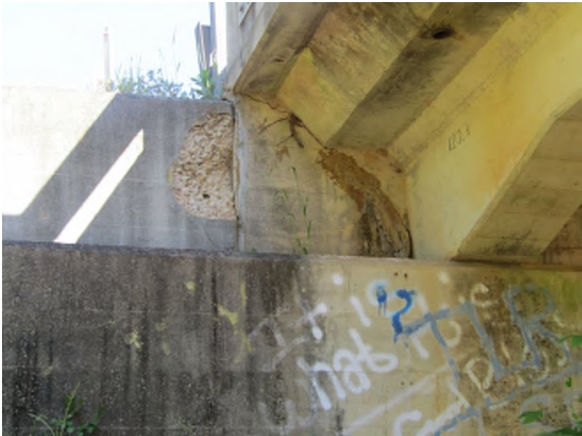
PHOTO 10 General Description endwall spalled
