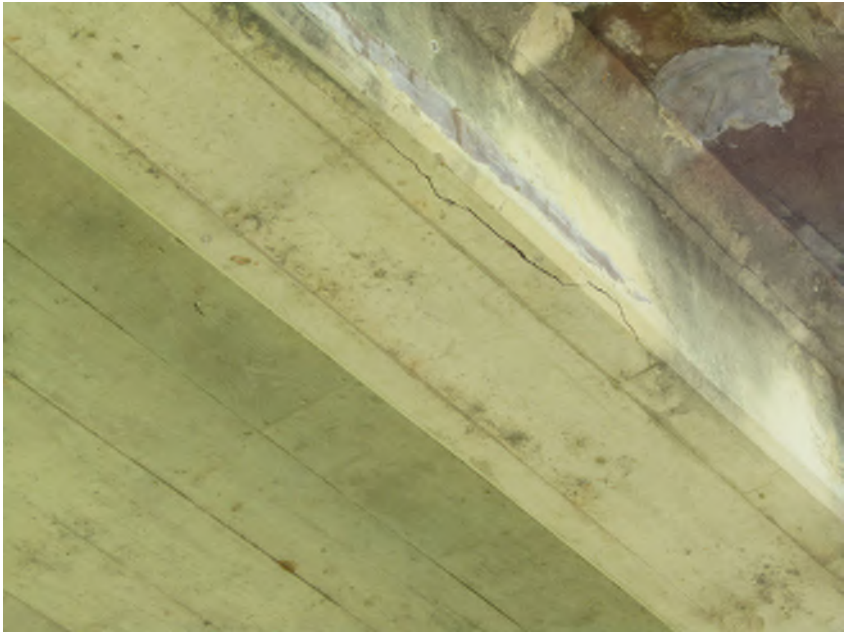
PHOTO 5 General Description horizontal crack in beam
